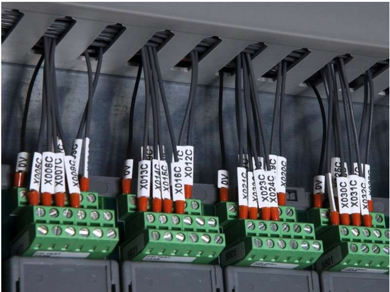
Figure 5 - Field Wiring Connections
