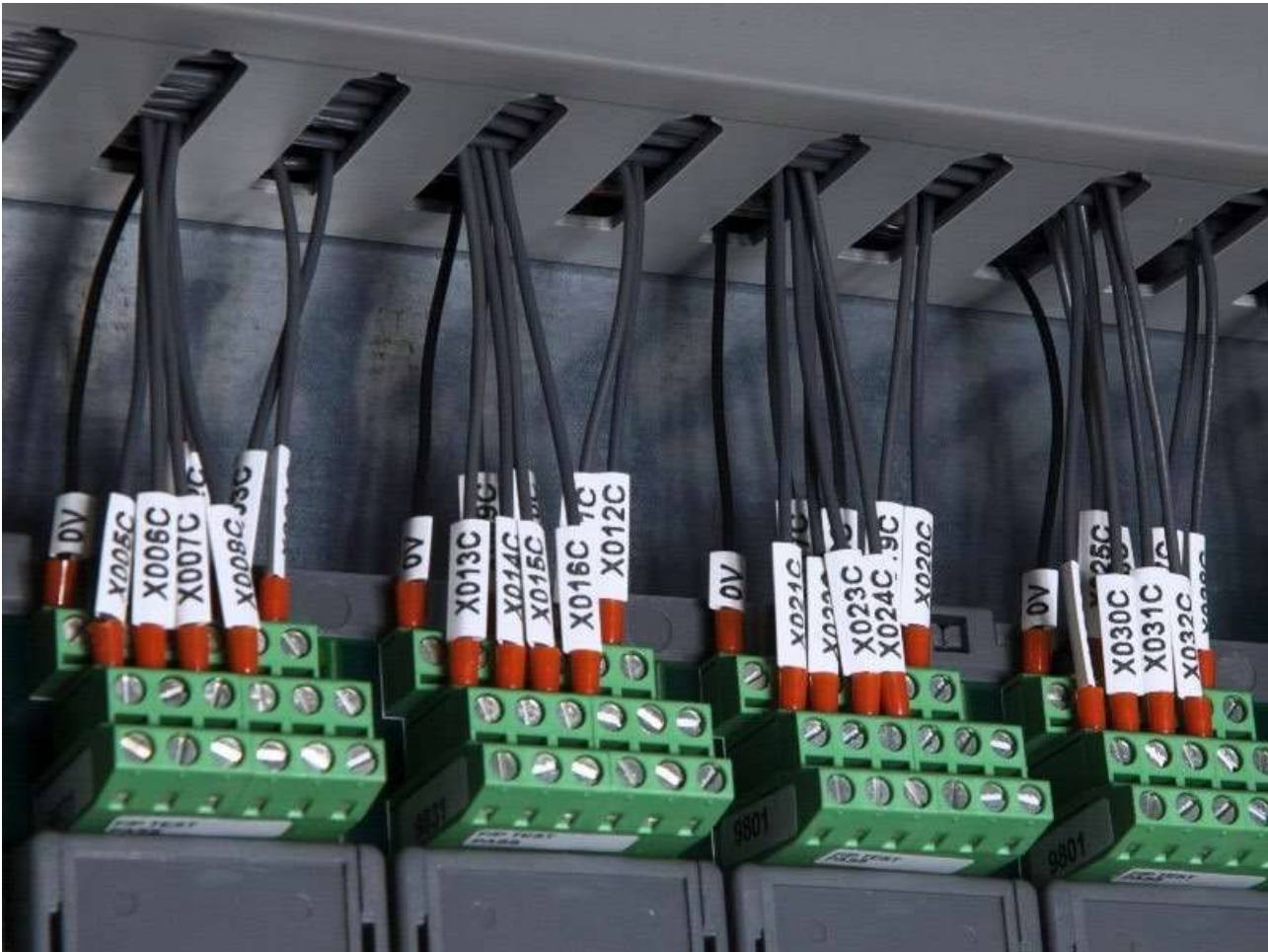
Figure 13 - Field Wiring Connections
